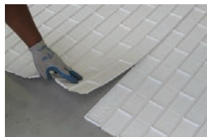
1. Lay Out Liner
