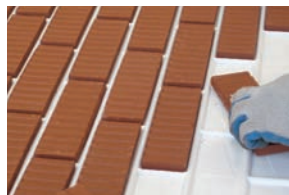
2. Install Thin Bricks
